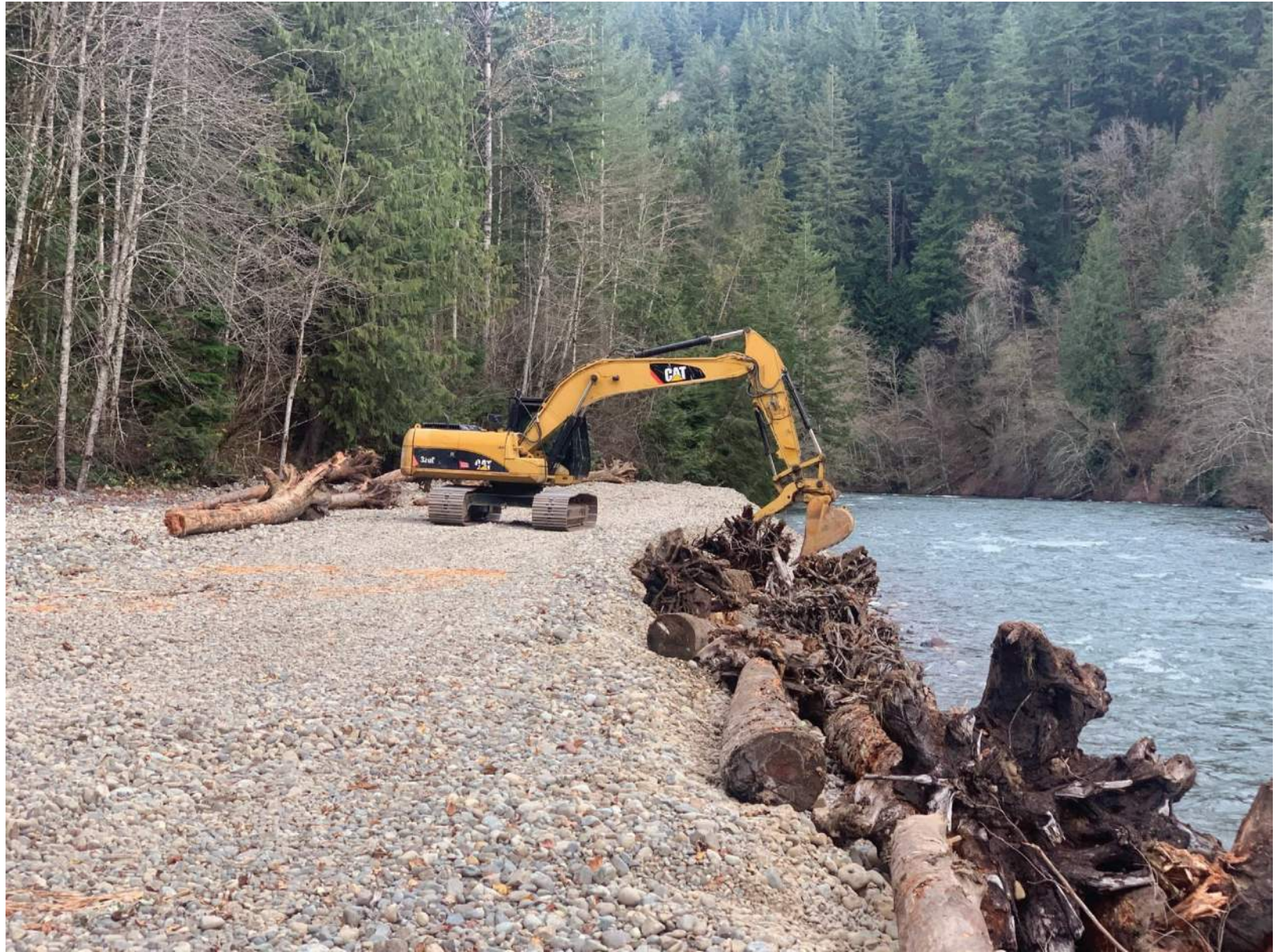
LWD stacking (18 NOV 2021)
