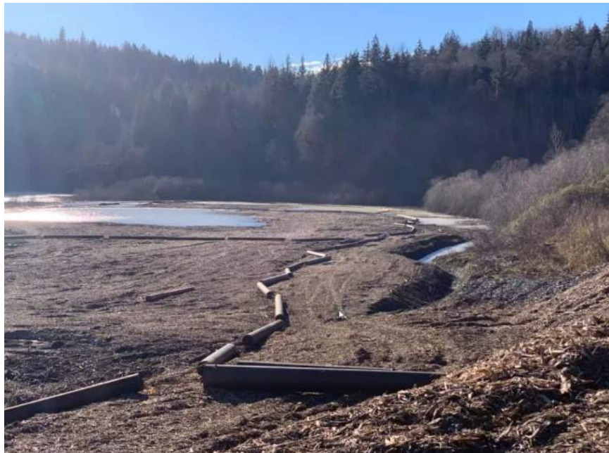
Photo 7-1. MMD Log Booms at Middle Basin
