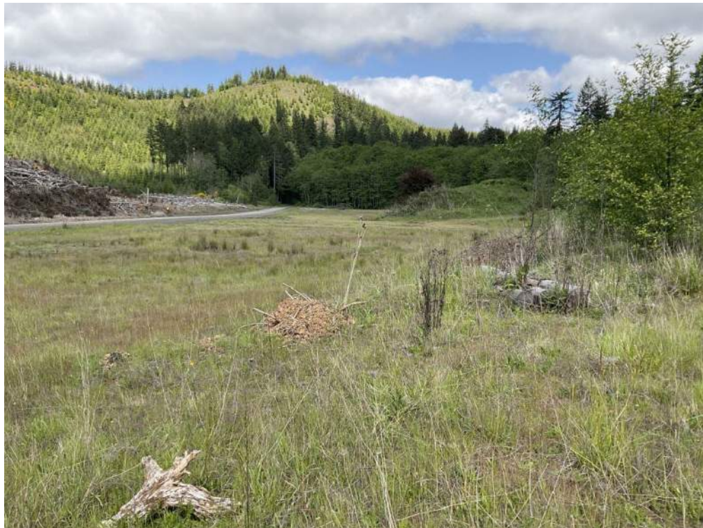
Photo 5-8. Cleared Eastern Side of Debris Storage Area C
