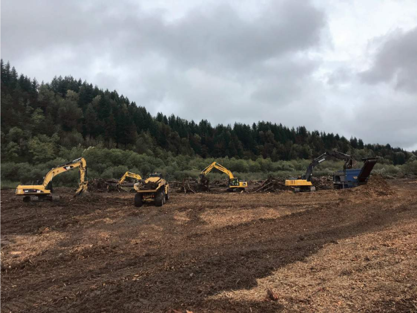
Chipping at the upper basin (2020)
